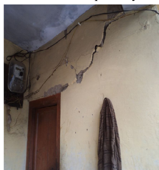
4c. Cracks on a wall
