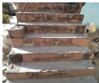
4f. Staircase beyond normal height of riser
