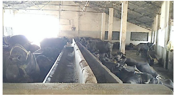
(b) Concrete structure, tin shed with feed alley in middle of the rows (face in)
