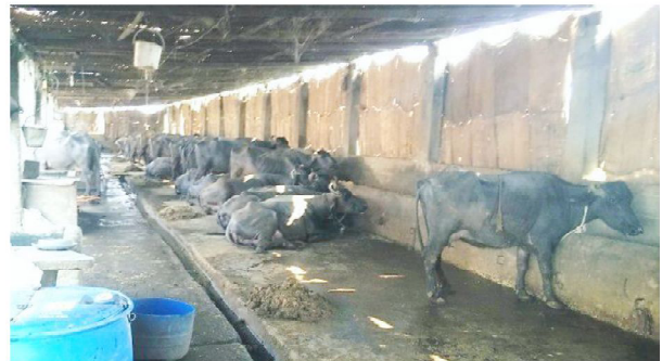
(h) Inner view of one side of dairy structure with feed alley at outer side and movement space for tractor in between two rows
