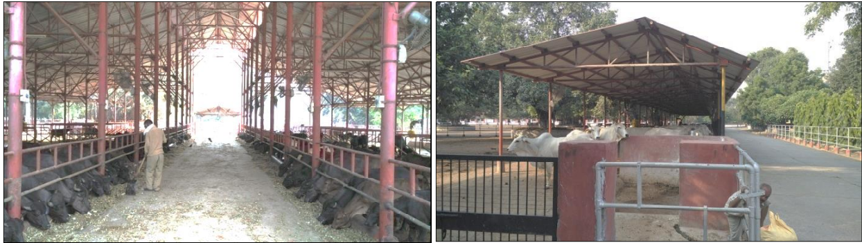
Fig. 2: A typical structure of dairy farm suitable for dairy mechanization at ICAR-NDRI Karnal
