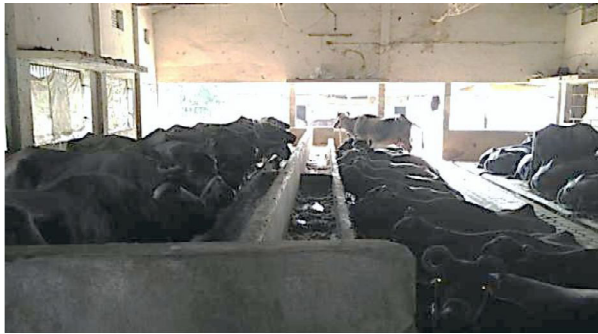
(a) Concrete structure, tin shed with feed alley in middle of the rows (face in)
